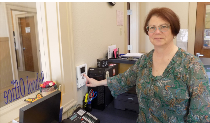
Office Manager Theresa Brumley demonstrates the remote access switch that allows her to see visitors before opening exterior doors.
